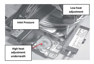
Check and adjust if necessary the valve inlet pressure after gas burner ignition
