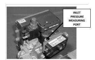
Check and adjust if necessary the valve inlet pressure after gas burner ignition
