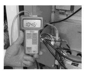
The out pressure must be measured on the pressure tap located on the gas injector support bar to avoid the pressure drop due to the elbow after the valve
